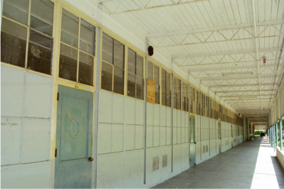
Figure 4: Side view of Classroom Building
