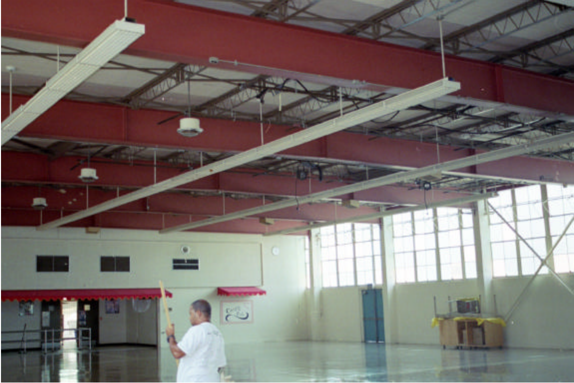
Figure 15: Cafeteria braced frames and roof framing
