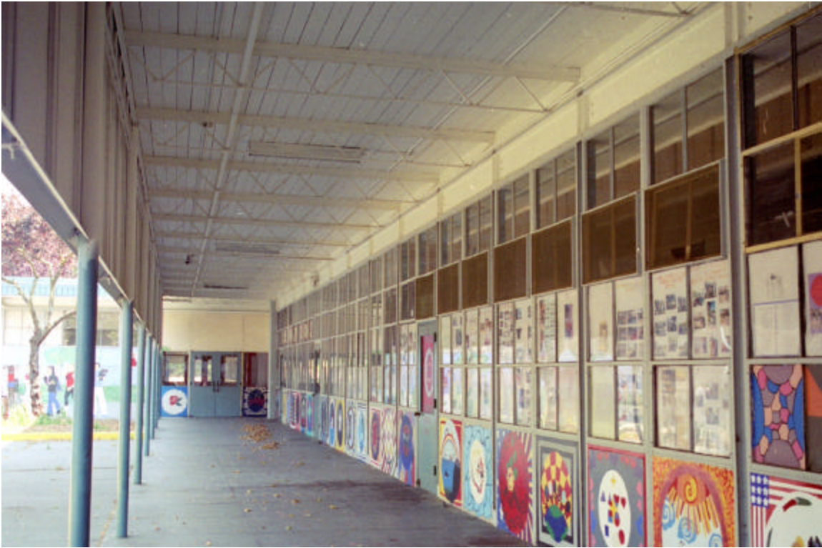
Figure 3: Side view of Classroom Building
