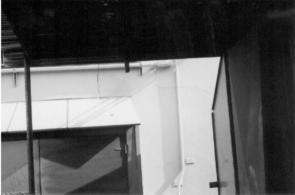
Figure 10: Cracks in the west wood-framed end wall of the Shop Building
