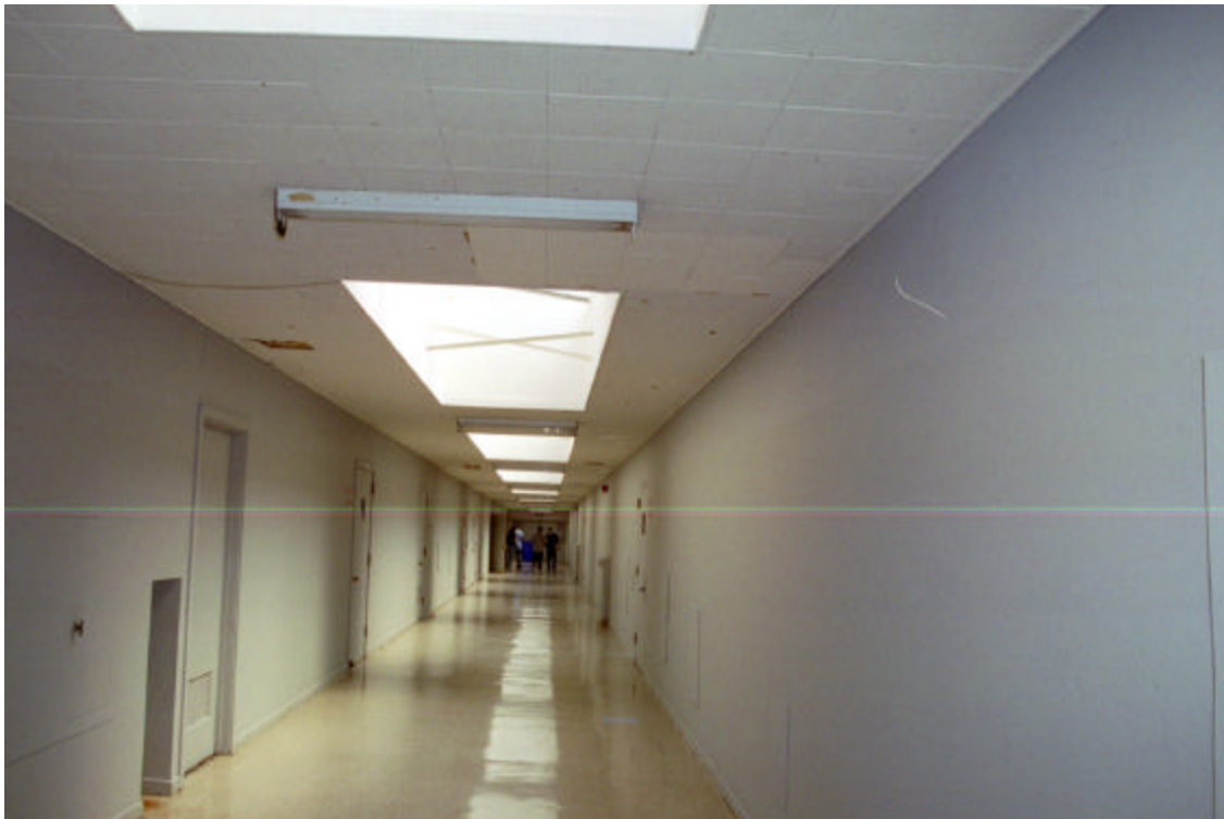
Figure 11: Diagonal bracing at corridor skylights in the Shop Building
