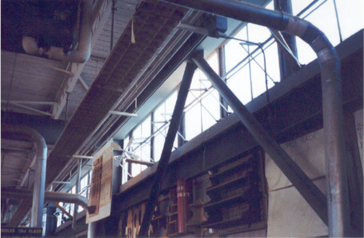
Figure 12: Braced frame at the Shop Building interior
