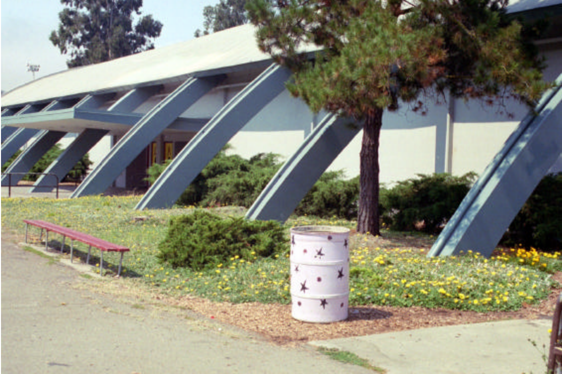
Figure 17: Buttresses at Gymnasium
