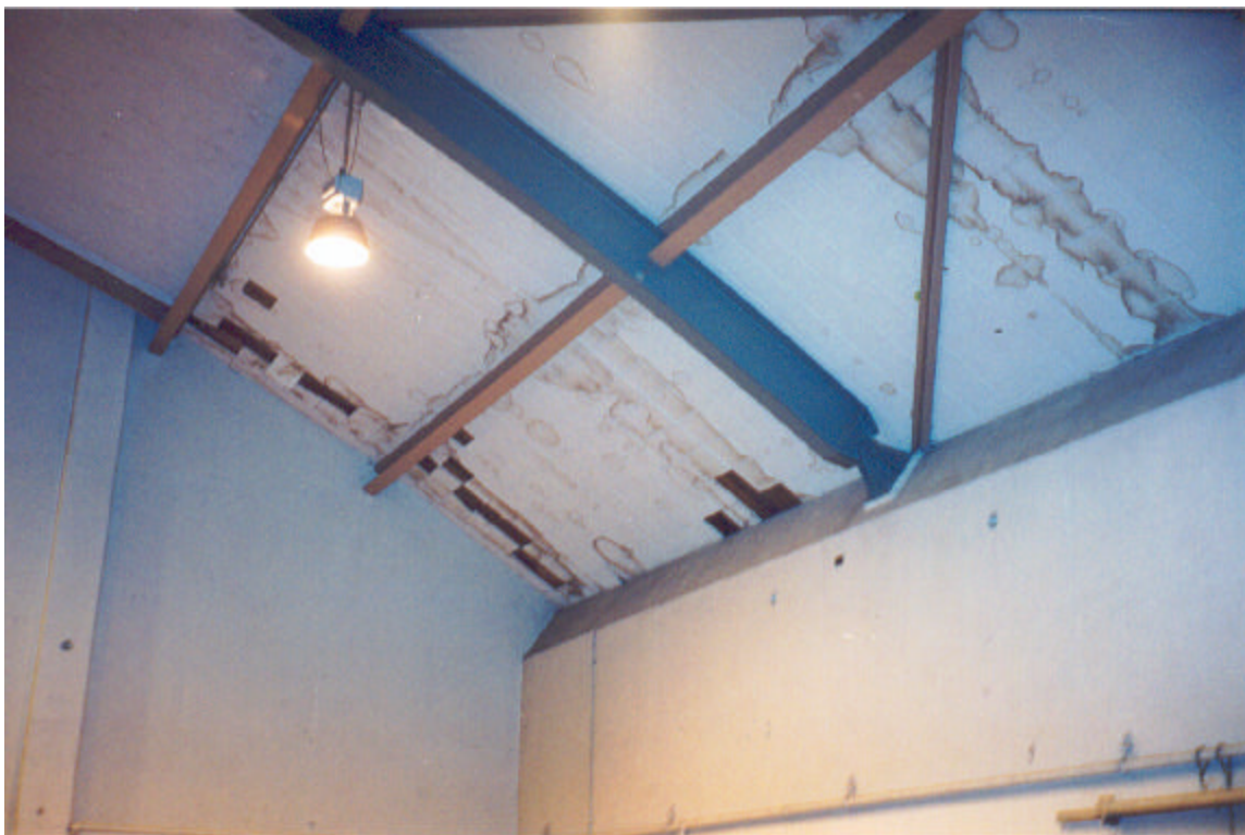
Figure 19: Water damage at the vaulted ceiling in the Gymnasium
