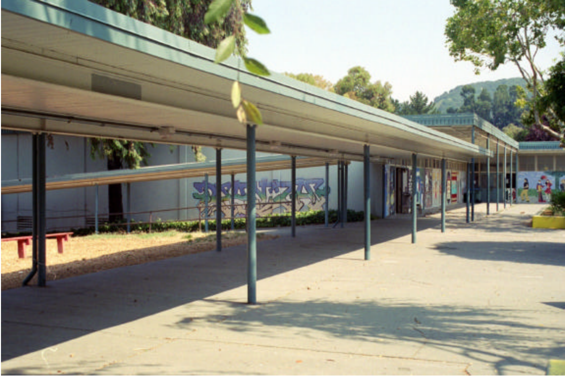
Figure 23: Covered walkway, typical
