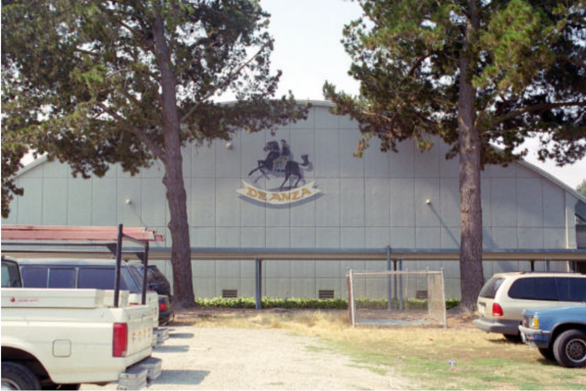
Figure 2: East side of Gymnasium Building
