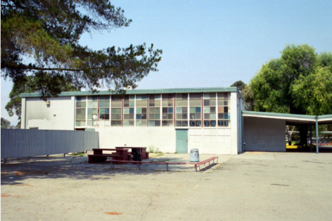
Figure 16: South wall of Cafeteria
