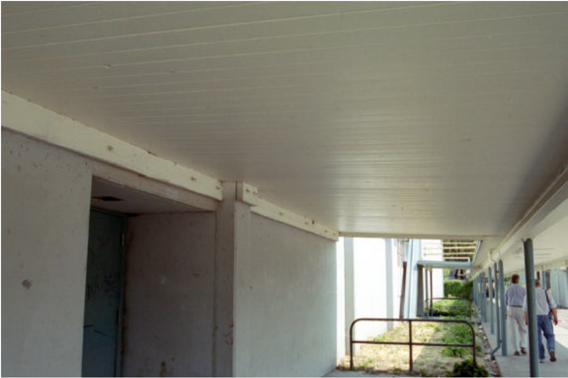
Figure 24: Ledger connection of covered walkway to locker room
