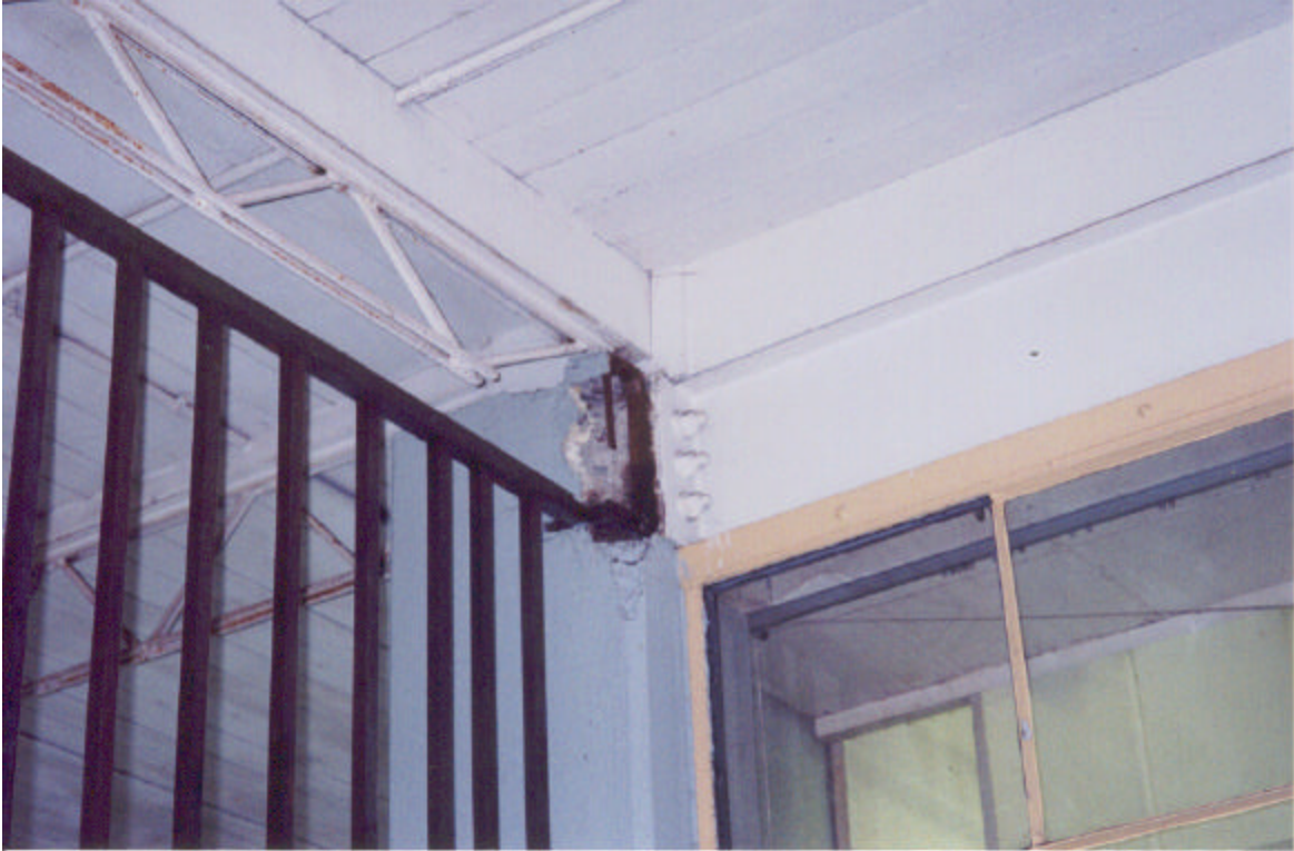
Figure 5: Cracking at truss support pilaster at Classroom Building, typical
