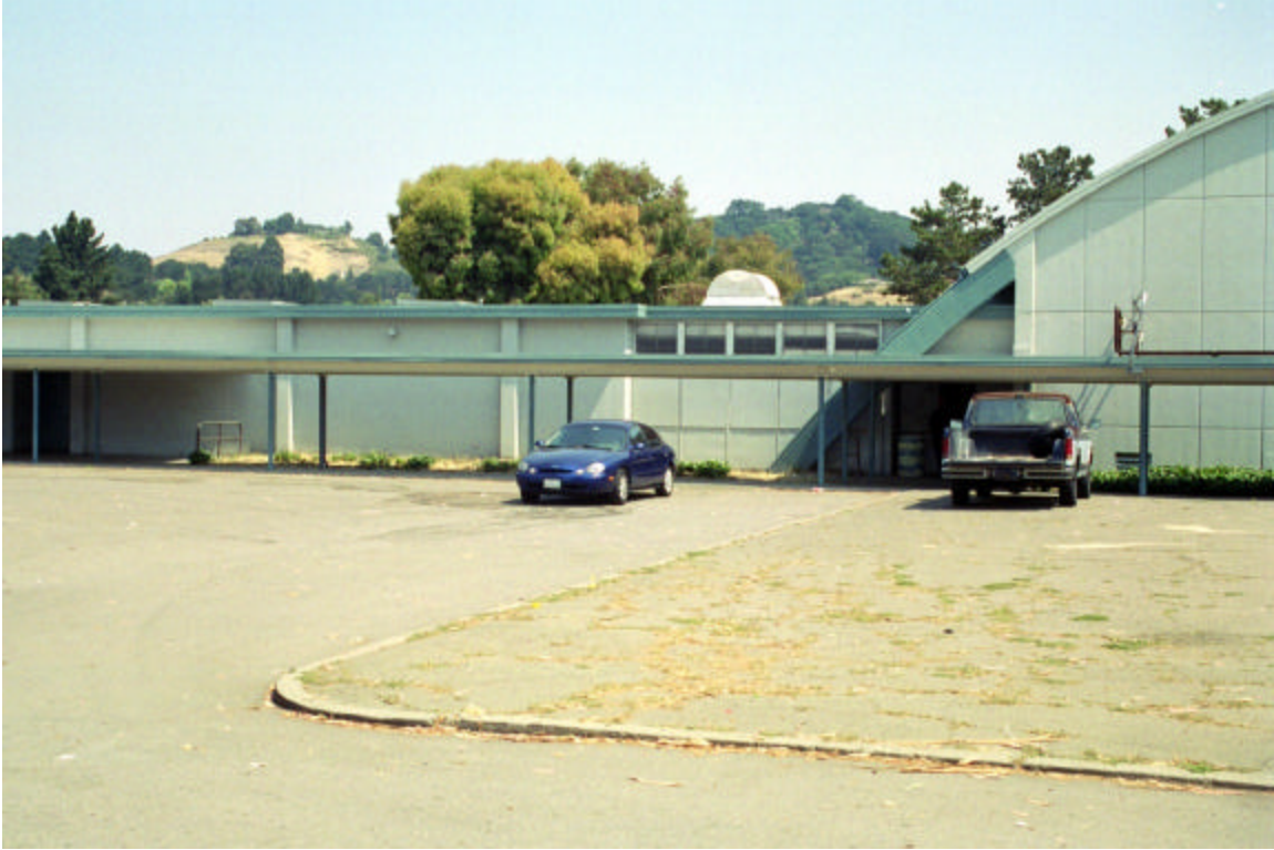
Figure 20: West side of Gymnasium and locker rooms
