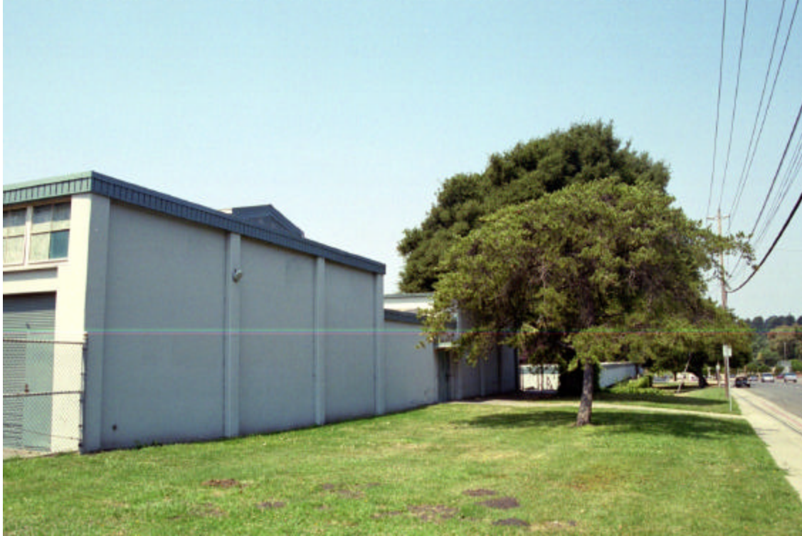
Figure 8: East end of Shop Building
