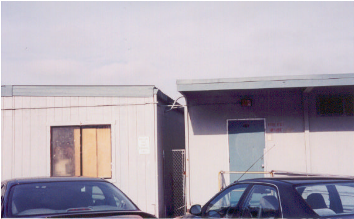
Figure 27: Conduit running between portable classrooms, typical
