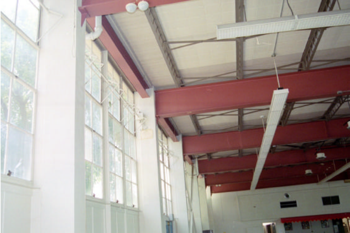
Figure 14: Cafeteria braced frames and roof framing
