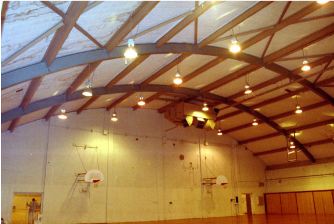
Figure 18: Vaulted ceiling in the Gymnasium
