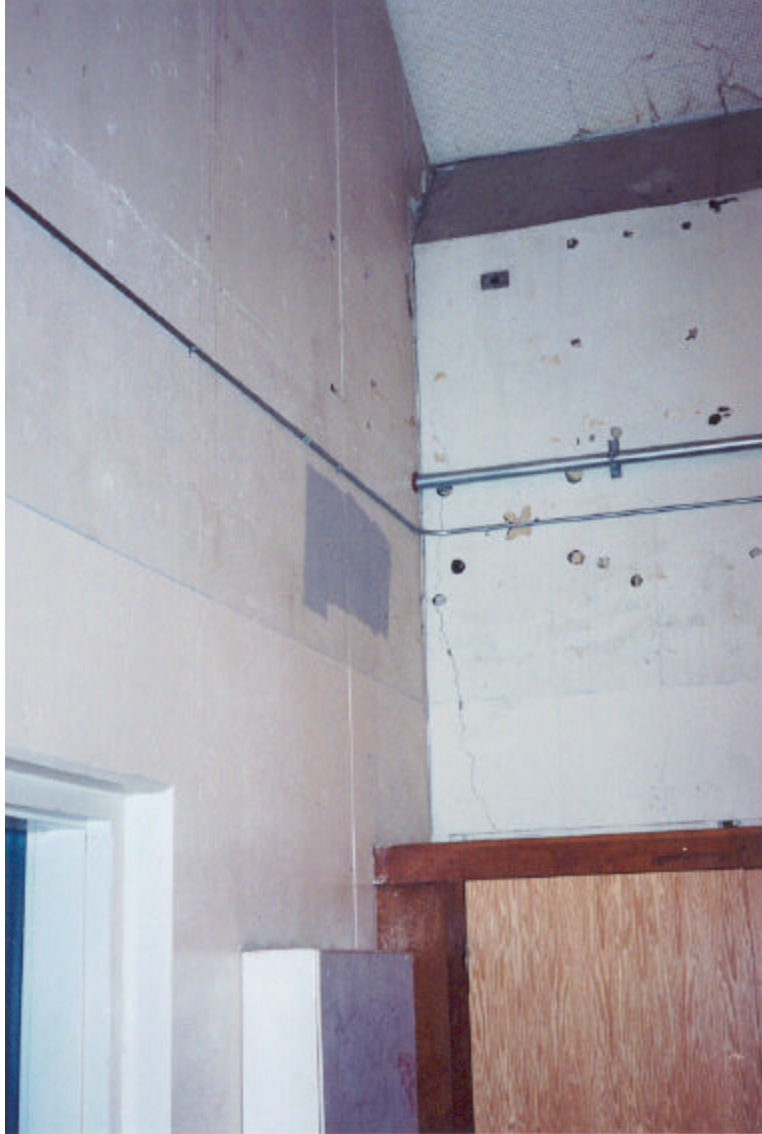
Figure 22: Cracks in the Gymnasium walls, typical
