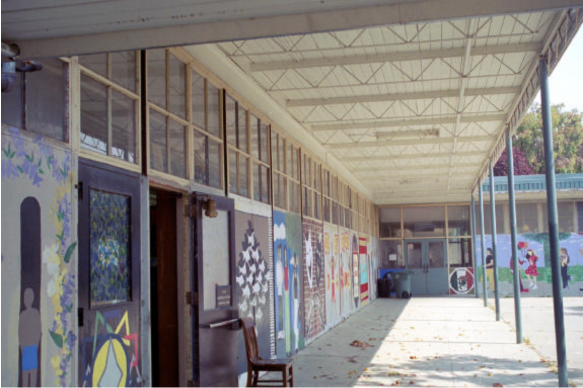
Figure 6: View of Classroom Building from courtyard
