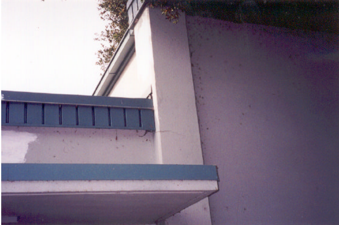
Figure 9: Cracks in the east concrete end wall of the Shop Building
